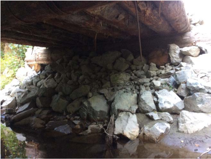
Right Bank Abutment when facing downstream
