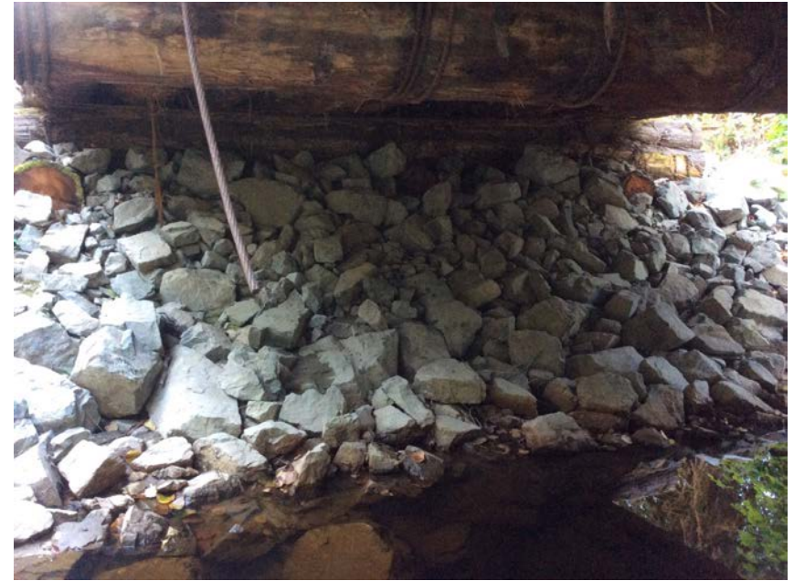
Left Bank Abutment when facing downstream
