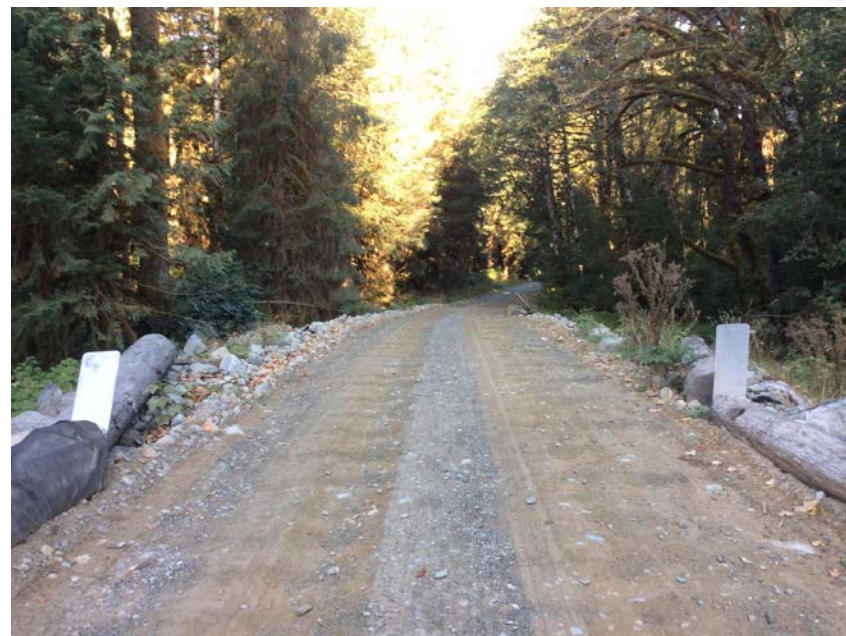
Right approach viewed from bridge
