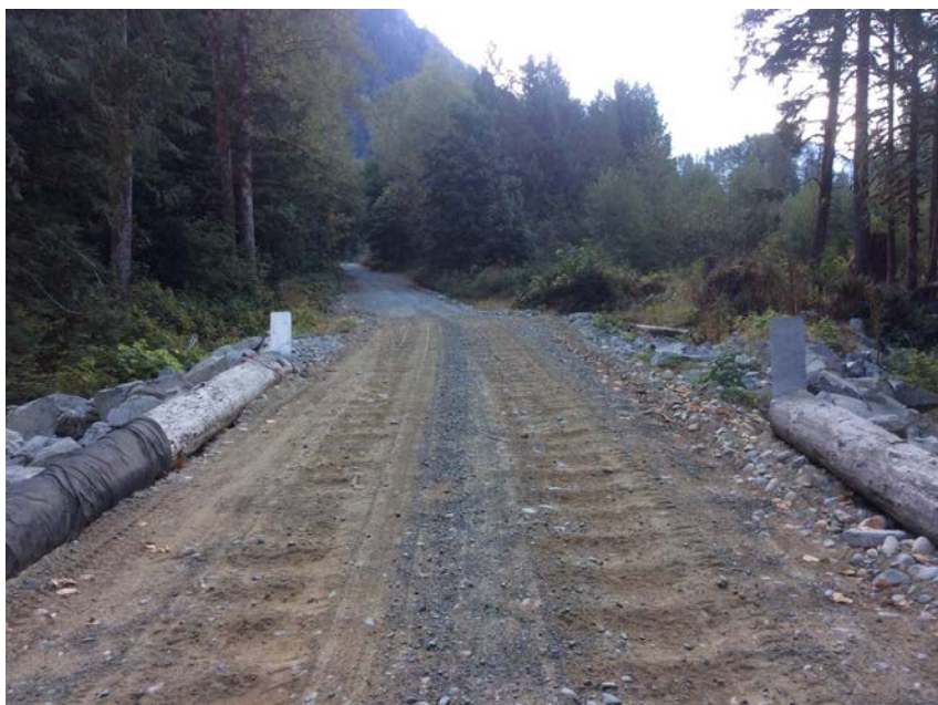
Left approach viewed from bridge
